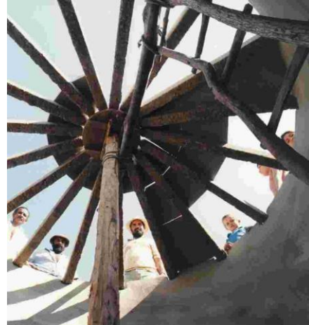
Illustration 2: Process of covering the cistern (inside view)
