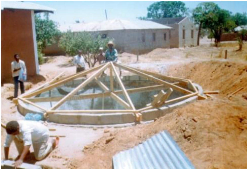
Figure 2: Construction of 52,000 litre sub-surface tank at Nzega town
