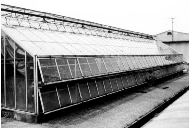
Photo 1 Greenhouse and gutter
