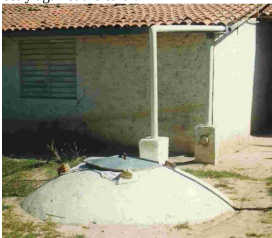
Illustration 7: Underground lime and bricks cistern
