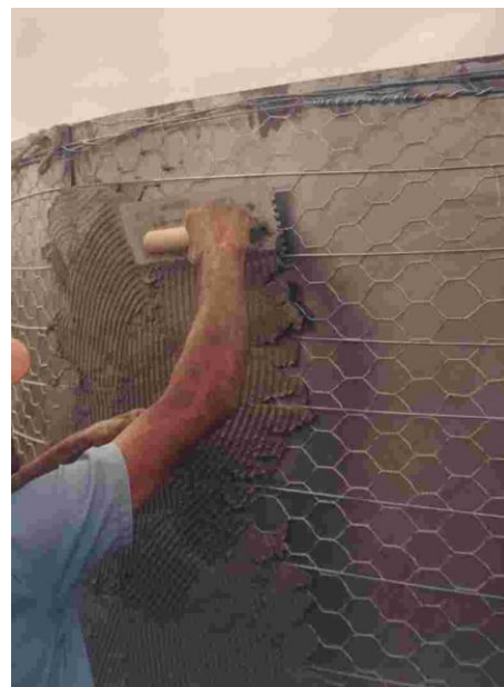
Illustration 6: Application of the first layer of mortar on top of the wiring
