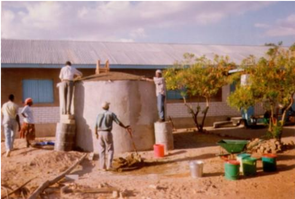
Figure 1: Construction of a 20,000 litre ferrocement tank at Lulumba Secondary School, Iramba district
